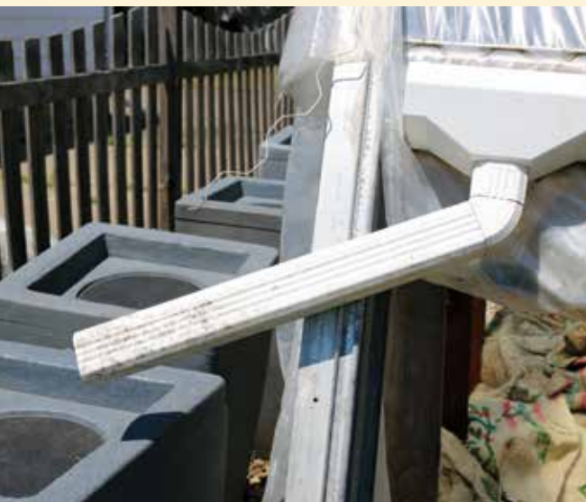
The rainwater harvesting system that Cherry Flowers and Tim Page added to one of the high tunnels at their urban farm in Minnesota. Photo by Marie Flanagan, North Central SARE
